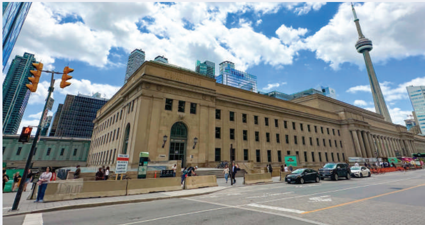
CURRENT STATE OF THE SECURITY BARRIERS.
