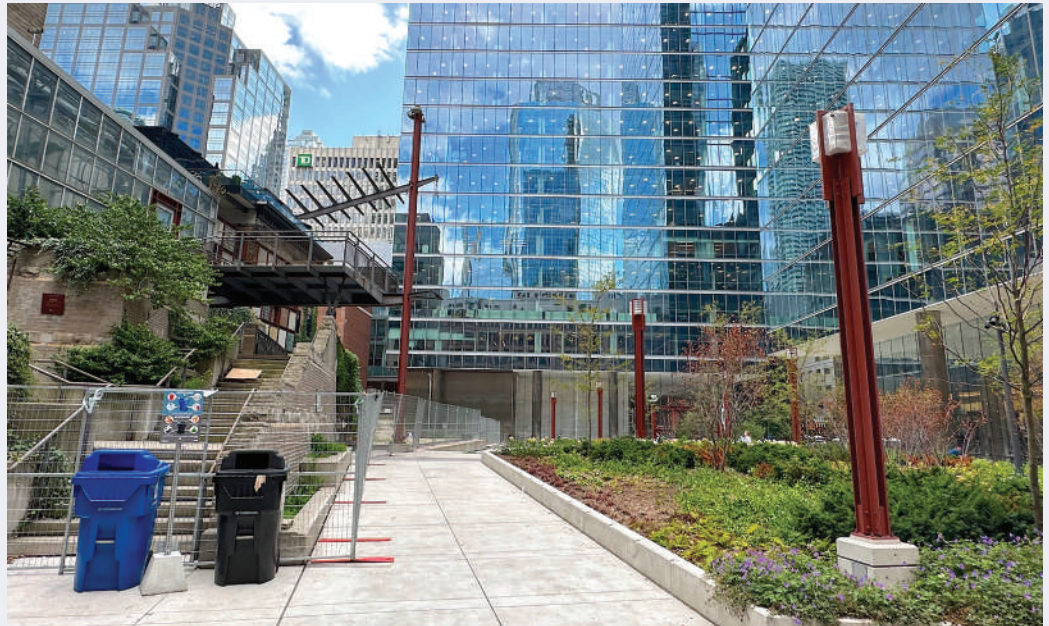
CLOUD GARDENS PARK HAS BEEN OPENED TO THE PUBLIC. HOWEVER, THE CONSERVATORY REMAINS CLOSED AND IN NEED OF REPAIR.
