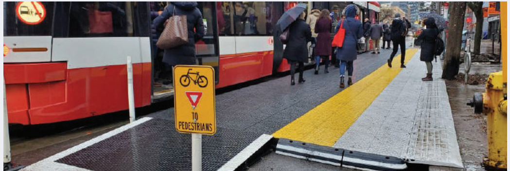
COMBINED BIKE LANE AND LOADING ZONE AT KING STREET & PORTLAND STREET THAT THE CITY IS TESTING TO REPLACE TEMPORARY KING STREET-CAR STOP INSTALLATIONS.
