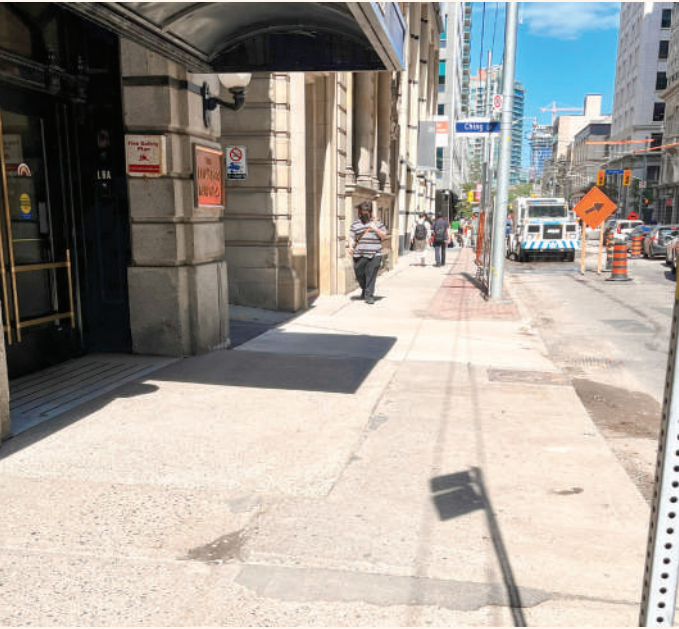
INCONSISTENT USE OF CITY STANDARDS MAKES STREETS APPEAR HAPHAZARD AND UNKEMPT AND ARE A FREQUENT SOURCE OF TRIP HAZARDS.
