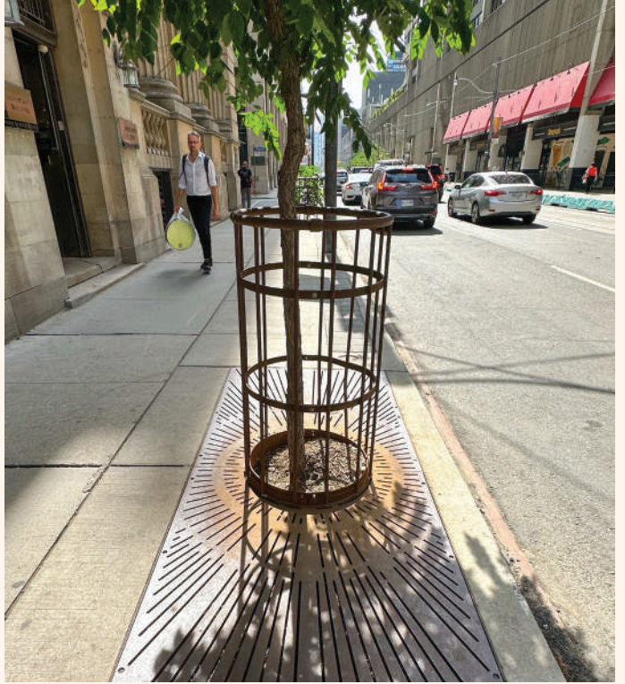
WEATHERING (“COR-TEN”)-STEEL TREE GRATES AND GUARDS ARE CORROSION-RESISTANT AND HELP PROTECT TREES FROM DAMAGE
