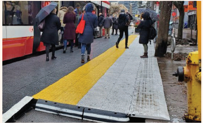
COMBINED BIKE LANE AND PASSENGER LOADING ZONE AT KING AND PORTLAND STREETS.
