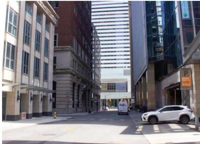
SHEPPARD STREET'S PERPETUAL SHADE AND NARROW SIDEWALKS MINIMIZE OPPORTUNITIES FOR IMPROVED TREE DETAILS. SHEPPARD STREET FACING SOUTH FROM RICHMOND STREET.
