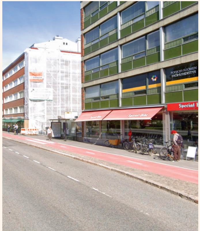
OULU, FINLAND'S LOADING PLATFORMS ARE INTEGRATED INTO RAISED CYCLE LANES COMBINED WITH THE SIDEWALK. THIS ALLOWS FOR LEVEL BOARDING AND HELPS KEEP SNOW OUT OF THE WAITING AREA.
