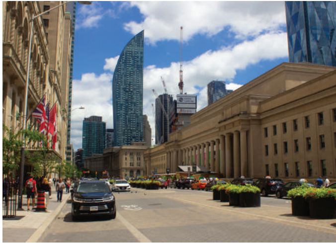
UNION STATION ON FRONT STREET IS A MAJOR GATEWAY TO THE FINANCIAL DISTRICT, WITH TAXIS OFTEN OCCUPYING BOTH CURB LANES. FRONT STREET FACING EAST NEAR YORK STREET.
