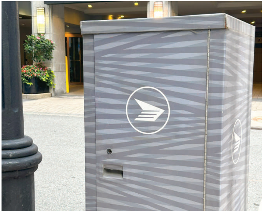
CUSTOM-DESIGNED GRAFFITI- AND POSTER-RESISTANT BELLA WRAPS HAVE BEEN INSTALLED ON POLES AND CANADA POST RELAY BOXES THROUGHOUT THE FINANCIAL DISTRICT. THEY ARE REPLACED EVERY FOUR YEARS TO AVOID DEGRADATION.
