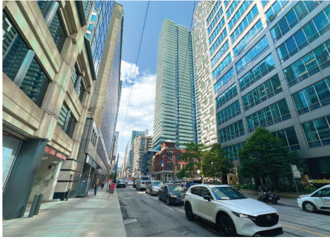
VICTORIA STREET'S PRIMARY FUNCTION DURING WEEKDAY BUSINESS HOURS IS OPERATIONS. VICTORIA STREET LOOKING NORTH FROM ADELAIDE STREET.
